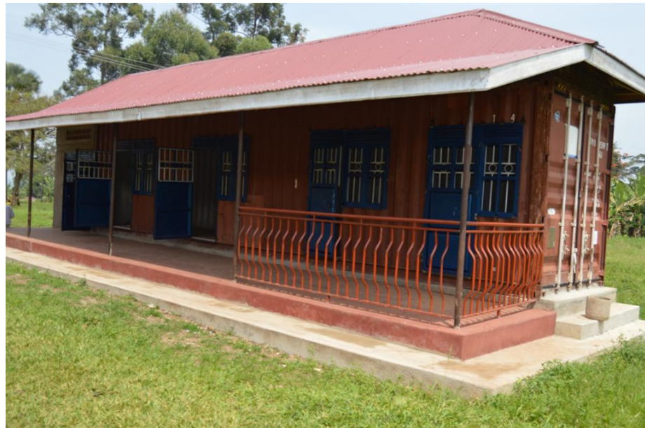
Windows and doors installed
