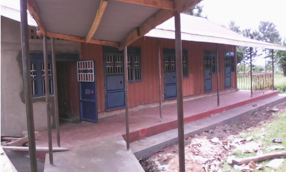
Side view after installation of windows and doors
