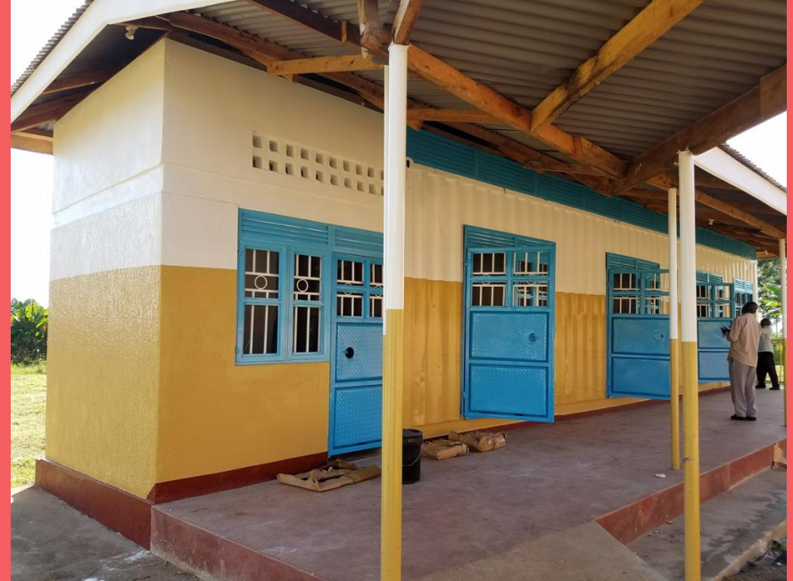
Side view of completed clinic
